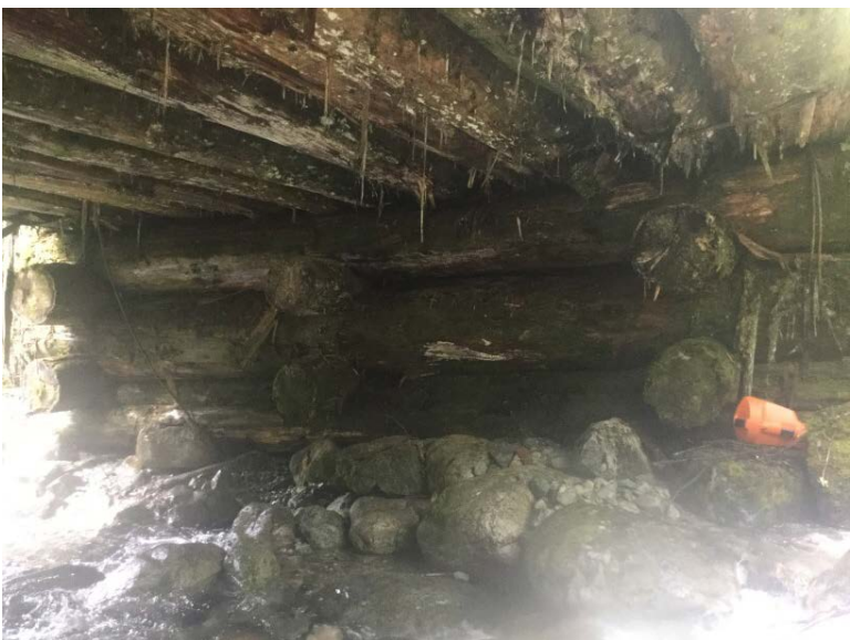
Right Bank Abutment when facing downstream
