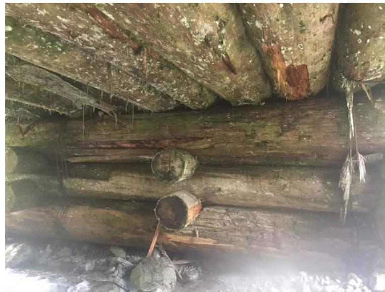
Left Bank Abutment when facing downstream
