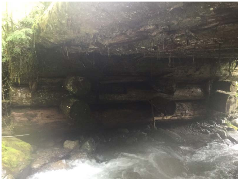
Left Bank Abutment when facing downstream
